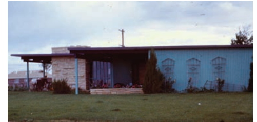
941 W. 99 th Avenue prior to a fire in 1962. (Photo by Donald Gravenstein)
